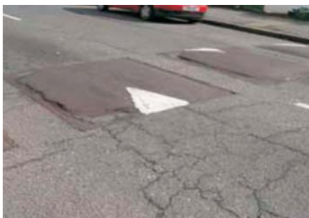
Potholes and differently coloured Surface may cause a loss of grip. (source: Craig Carey-Clinch, MCI, UK)
