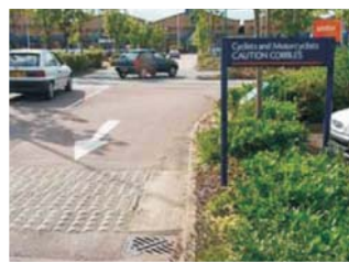
These speed inhibitors form a potential hazard for the rider because of the loss of grip on the surface (source: DTV Consultants, NL & C. Carey-Clinch, MCI)
