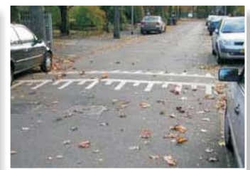
Speed inhibitors (speed bumps) form a small change in vertical alignment while maintaining surface grip, so can be safe for the PTW rider (source: DTV Consultants, the NL).
