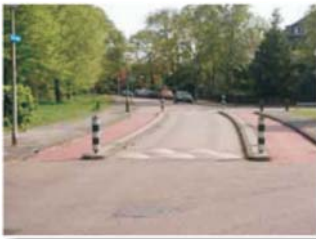
These speed inhibitors form a potential hazard for the rider because of the loss of grip on the surface (source: DTV Consultants, NL & C. Carey-Clinch, MCI)
