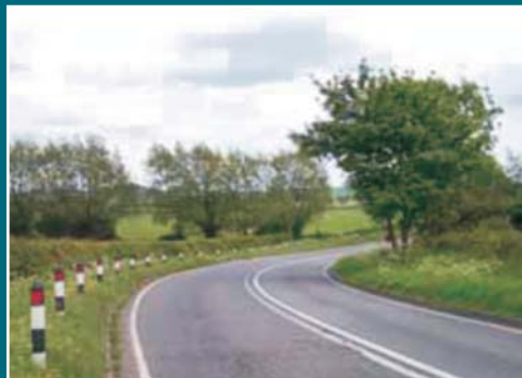
This bend has been fitted with marked posts to make it more predictable (source: A.J.Sharp IHIE)
